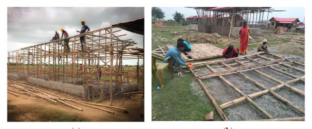
(a) (b) **Fig. 3**. CBFT construction in Nepal: (a) typical construction methodology; (b) Prefabricated CBFT construction.
